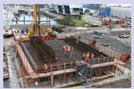
Figure 1 Selective use of stainless reinforcement on the pile cap of the 300 year life Gateway Bridge, Australia, specified by Aecom using predictive modelling. Courtesy of Outokumpu
